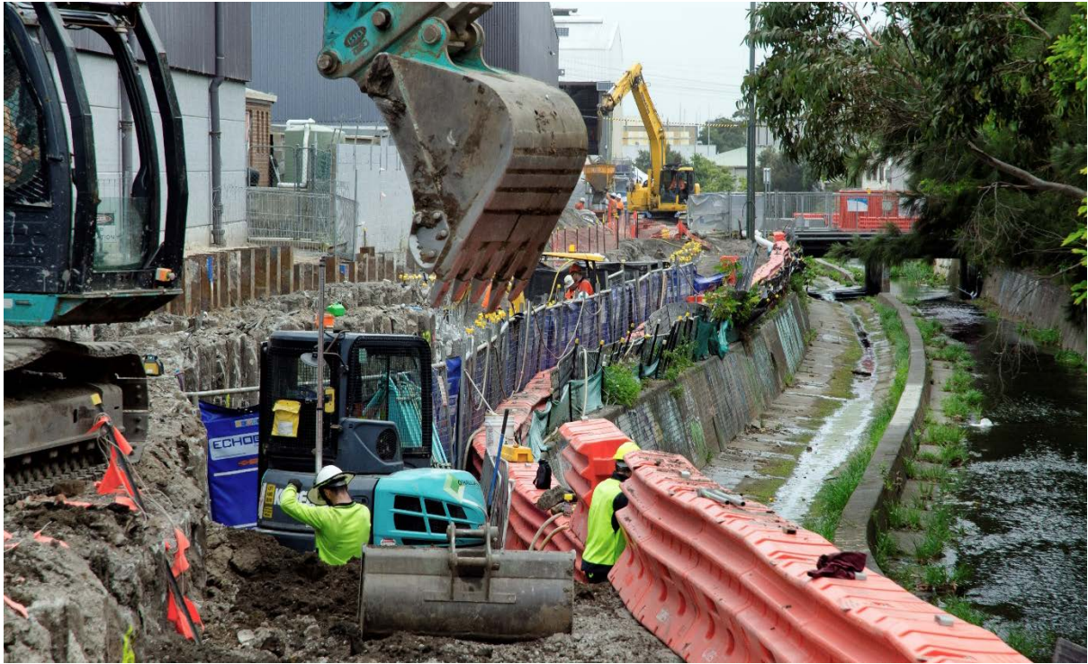
Widening of the open channel near Alexandra Canal
