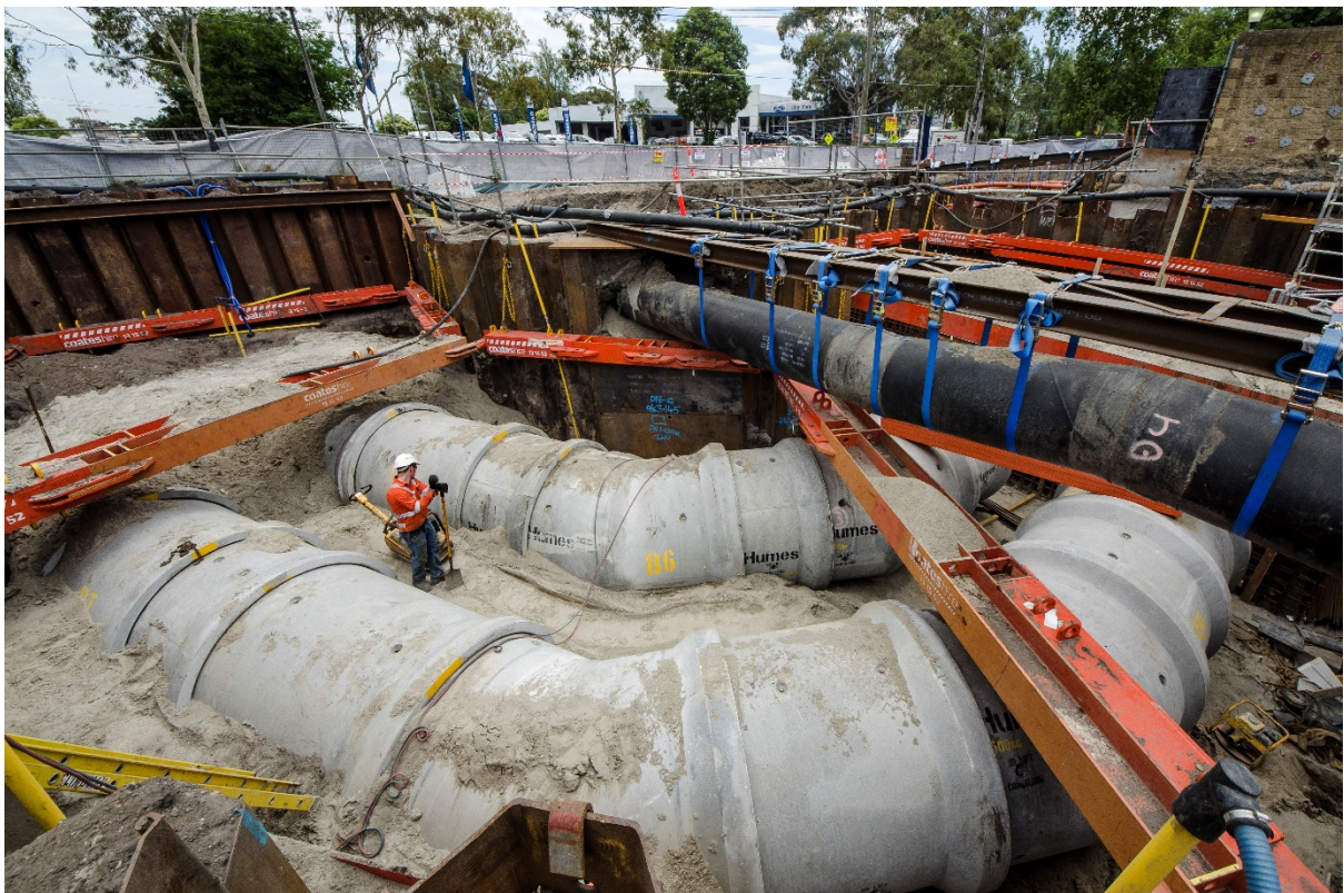
Connection to Joynton Avenue trunk drain
