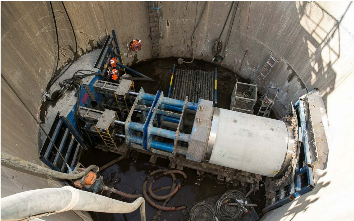
Micro-tunnelling and jacking pipes
