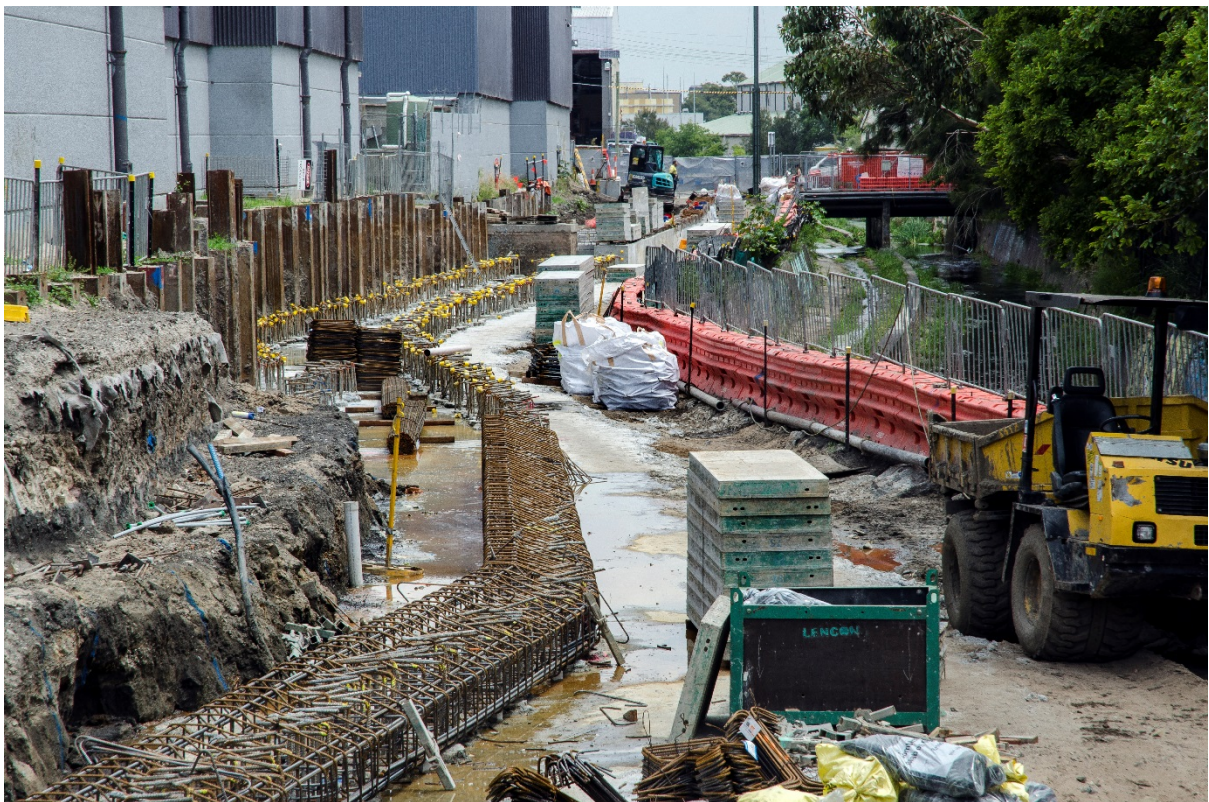
Widening of the open channel near Alexandra Canal
